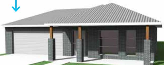
Two approaches to materials on a house
